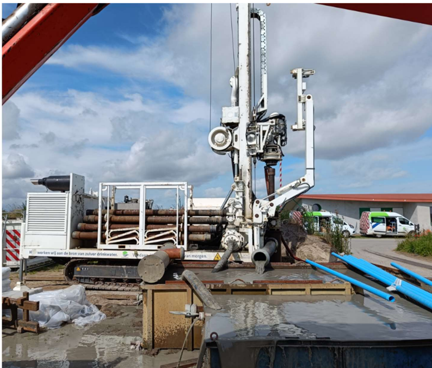
Figure 3.5: Drilling of monitoring well PPo/d.
